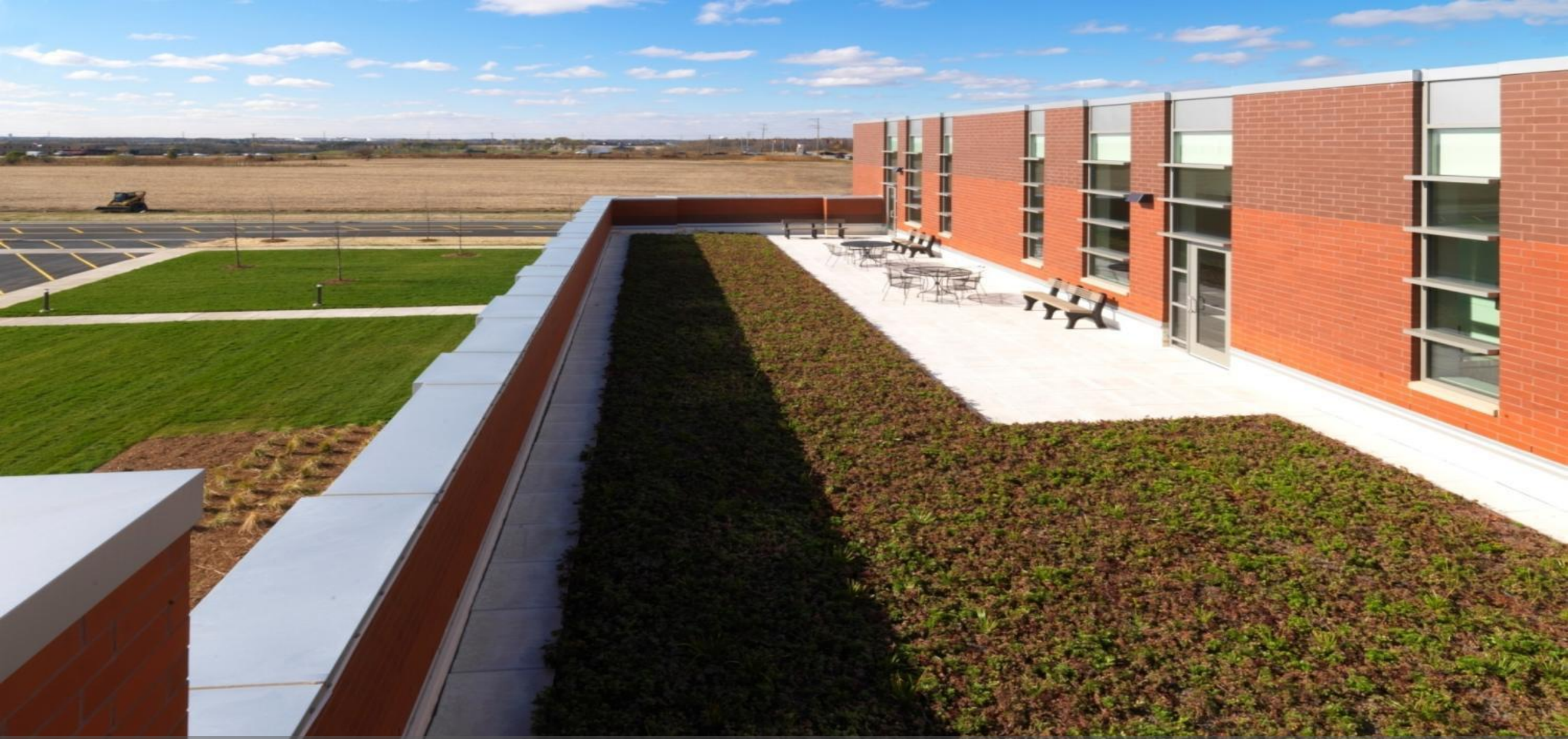
Moraine Valley Community College / Southwest Education Center / Accessible green roof garden and educational space
