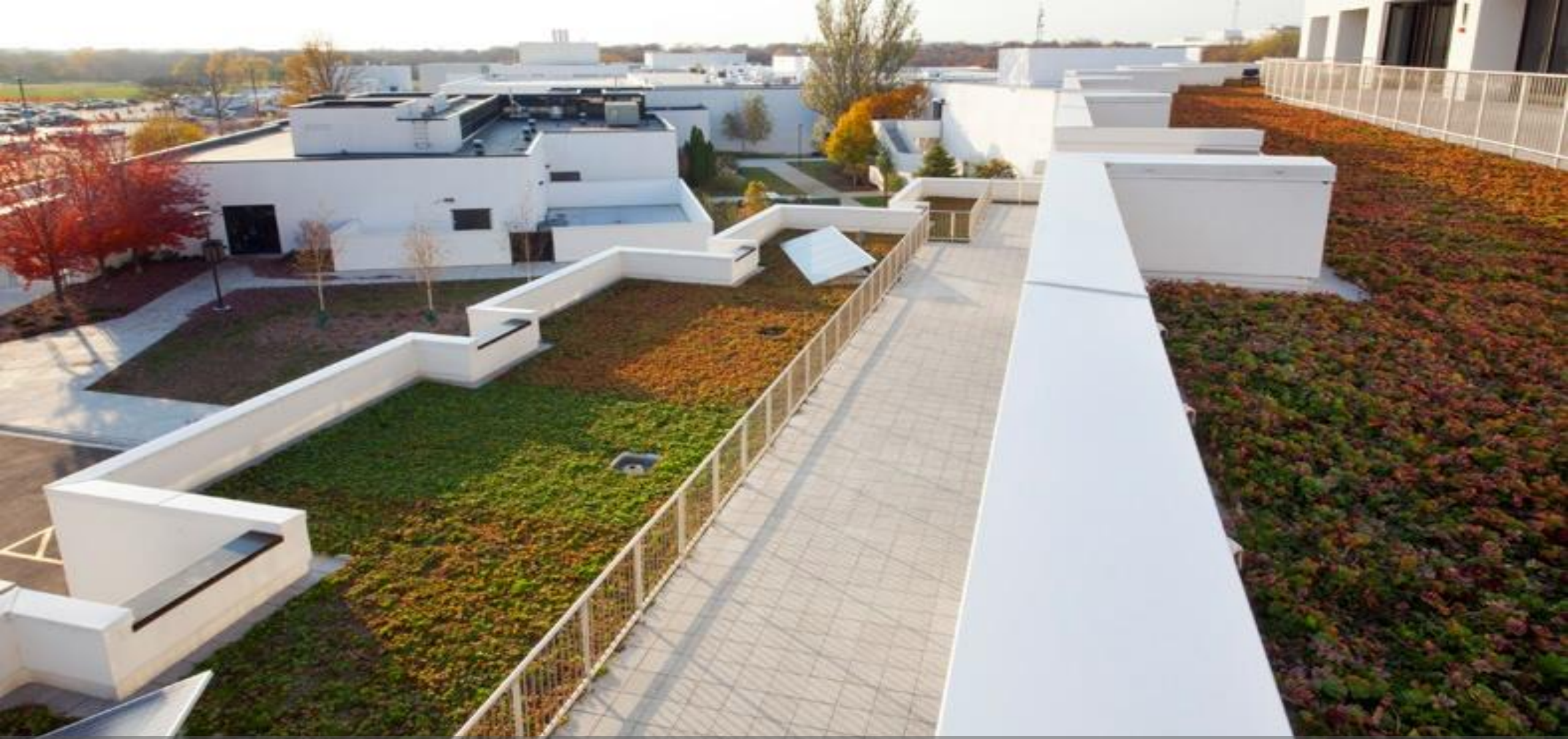
Joliet Junior Community College / Campus Center / Accessible green roof garden
