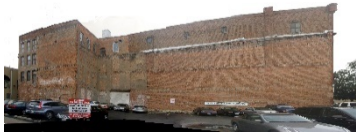
Demolition of Existing White Store
