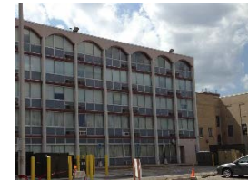
Demolition of Existing Hotel Building
