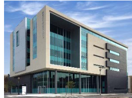
Complete Construction of Core & Shell
